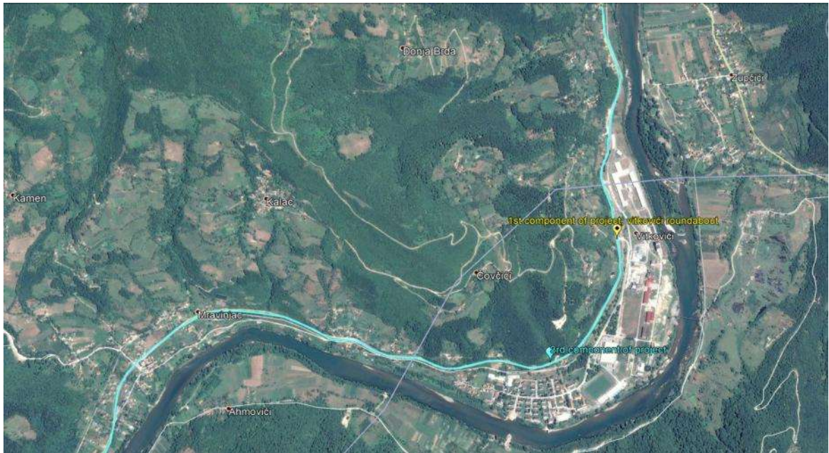
Figure 12: 3rd stretch of project, improvement of road section Ustikolina-Goražde
